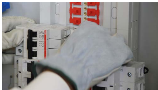
The Breaker Snaps Into The DIN Rail
