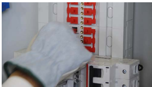
The Protective Cover Is Removed
