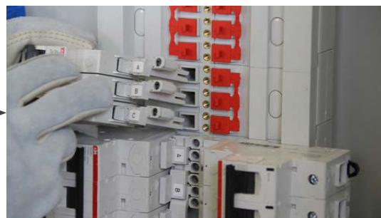
The Breaker Is Inserted Into The Opening
